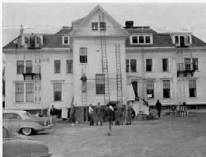
Finishing up the back of the house.
